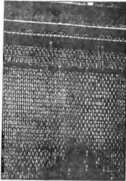
A double layer of polypropylene mesh is used as a collector in the Camanchaca Project in Chile. The fiber is 1 mm wide and 0.1 mm thick. The horizontal fibers in the weave are 1 cm apart.
