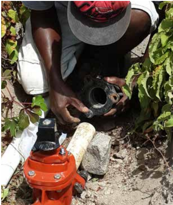
Installing a valve to ensure good control of water system.
