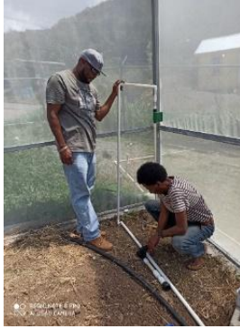
Plate 5: CARDI Technician installing drip irrigation in a Protected Agriculture system
