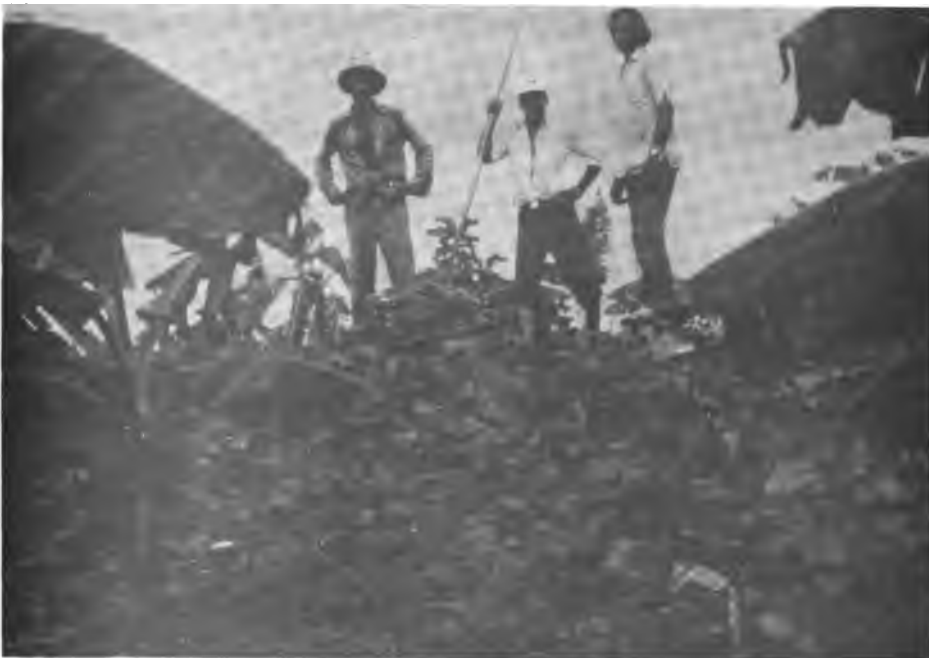
b) Farmers and the agricultural officer demonstrate the height of the dam after the drainage canal is cleared
