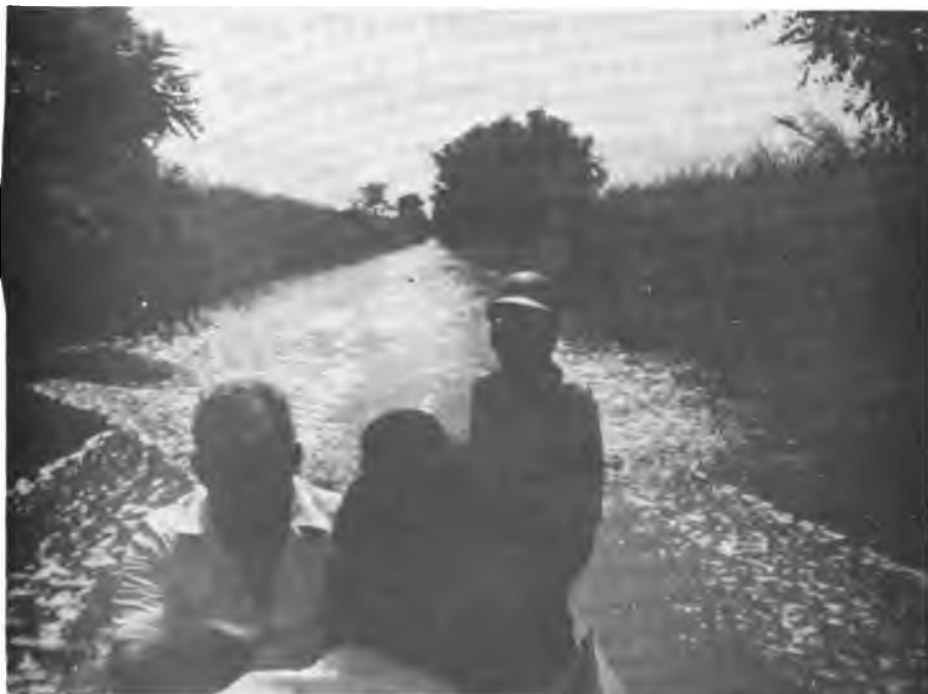
c) View of a drainage canal after the infrastructural works
