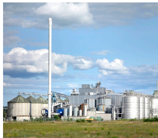
■ FIGURE 7. DISTILLERY PLANT
