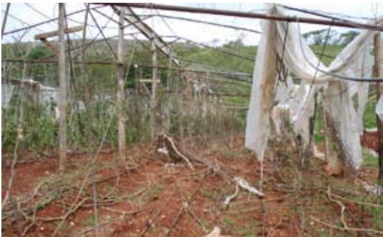
An example of the kind of damage caused by Hurricane Dean to 90% of the island's greenhouses.
