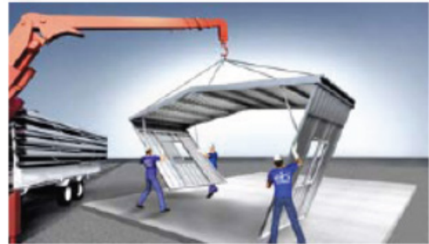
3 Abertura das paredes Opening of the walls
