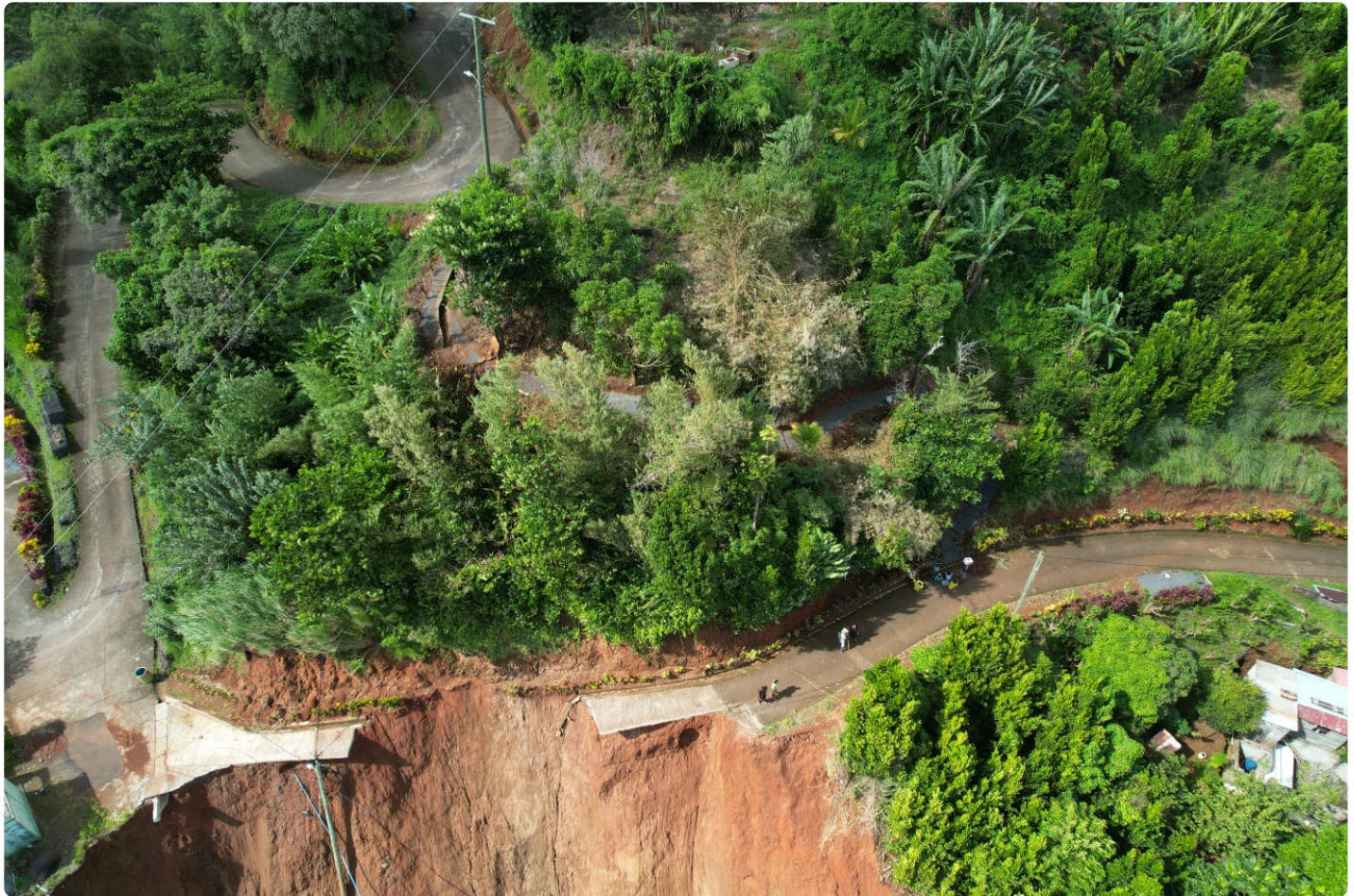
Drone image, showing the impact of landslides on physical infrastructure (Amos Benjamin)
